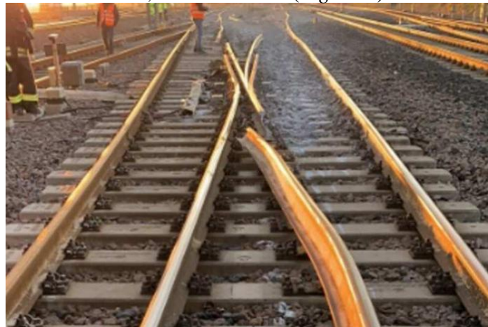
Figure 8 – Initial point of derailment: switch 05 at km 166+756 (source: web)
