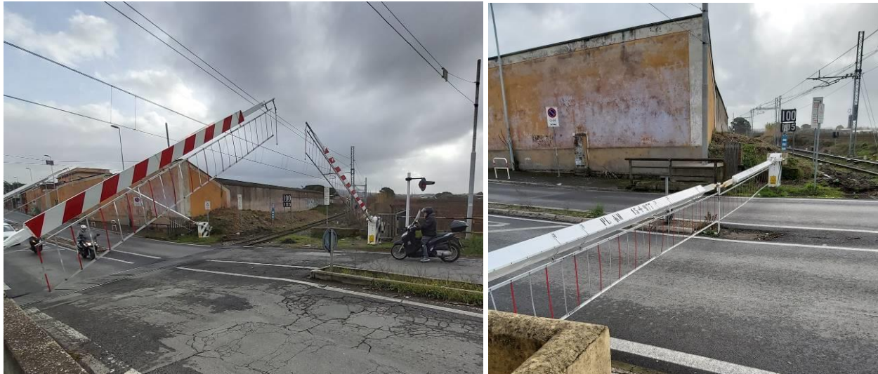
Figure 7 - Barriere del PL km 15+977 (fonte Digifema)
